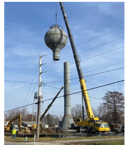
Nilwood – New elevated water tower
